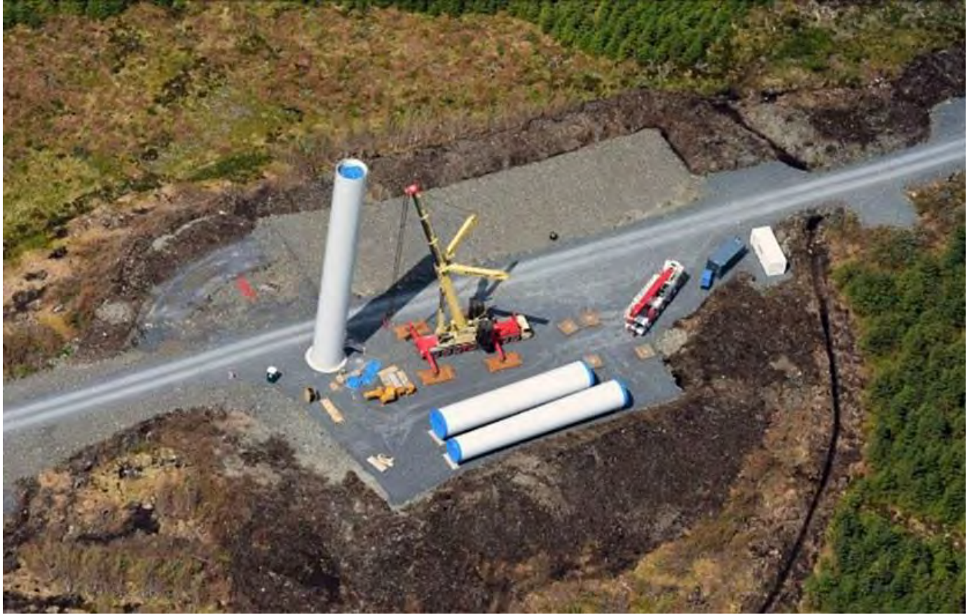
Above: Tower construction at SPR's Kilgallioch Windfarm
